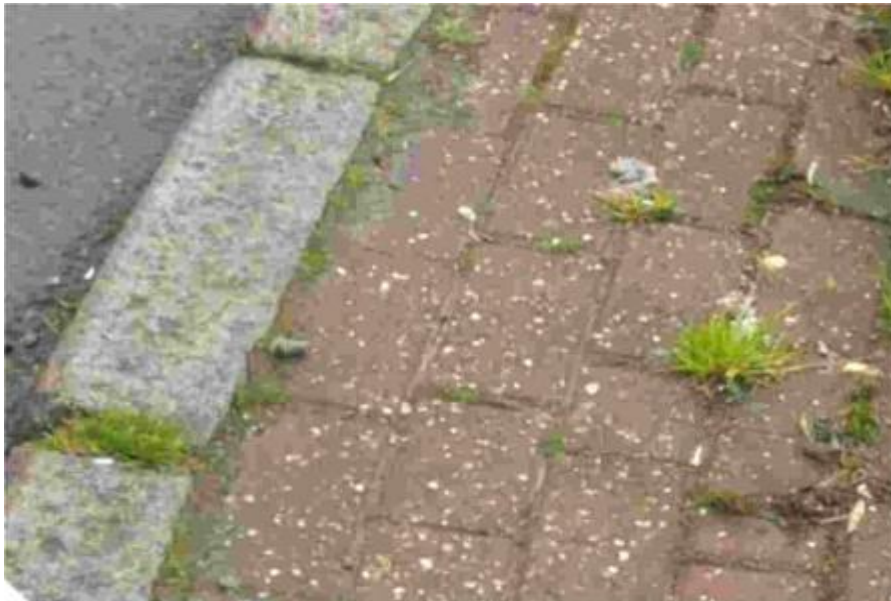
Paving is sound and the bricks intact. It just needs cleaning, weeding and re-pointing.
