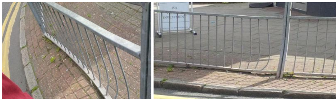
It is commonly known that without protection replacement railings at this corner get damaged by tightly cornering lorries. Just ask the locals.
